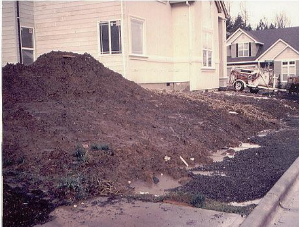
Figure 24 (a): Sidewalk Subgrade Gravel Barrier Figure 24 (b) sediment trap
