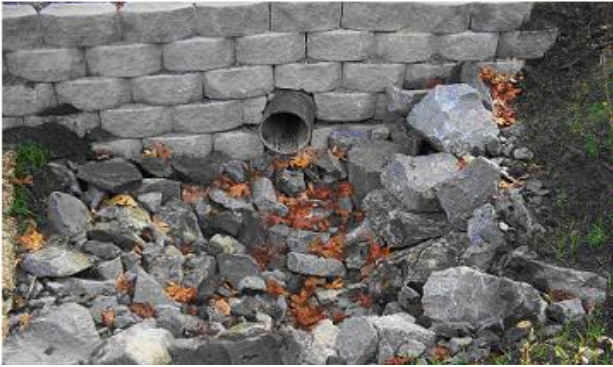
Figure 26: (c) Outlet protection
