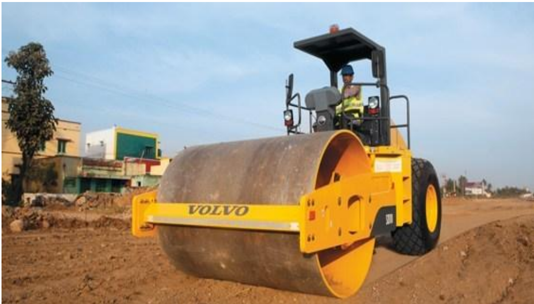
Figure27: Compaction of Soils (Using loader)
