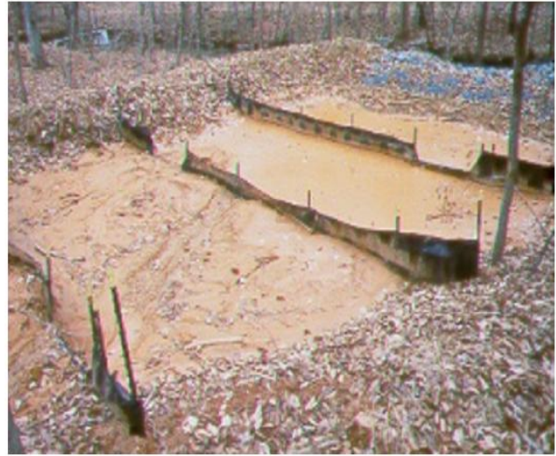
Figure 24 (a): Sidewalk Subgrade Gravel Barrier Figure 24 (b) sediment trap
