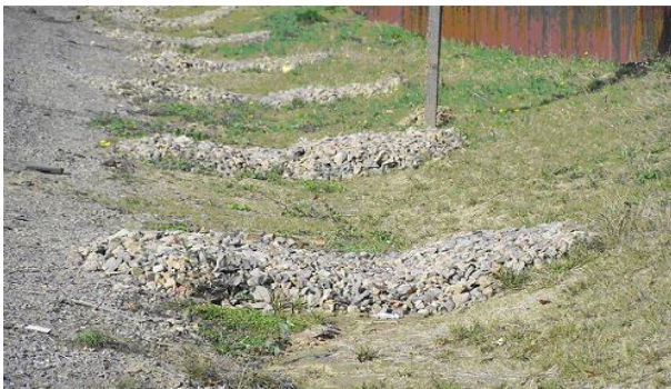
Figure 26: (a) Check dam
